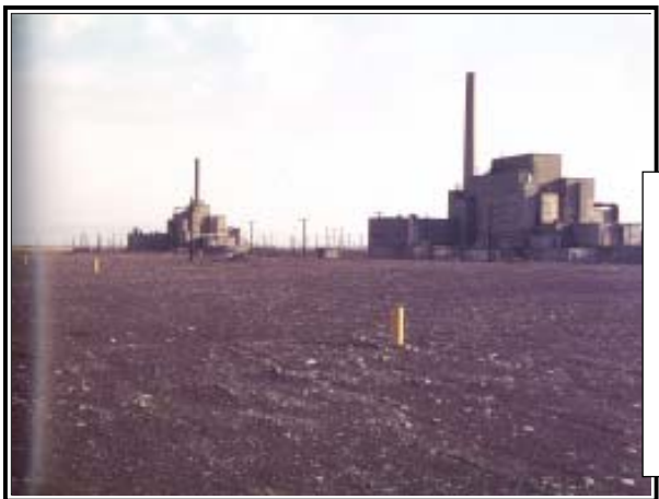
Nuclear Reactors D and DR [Hanford, Washington Site] These reactors are now decommissioned. D Reactor was one of the three original reactors built between 1943 and 1945. The R in DR stands for "replacement." The yellow posts identify buried radioactive waste and potential surface contamination. (p. 77)
